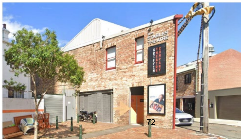
Photograph 2: Northern facade of the existing Stables Theatre, looking south (Source: TZG Architects)
